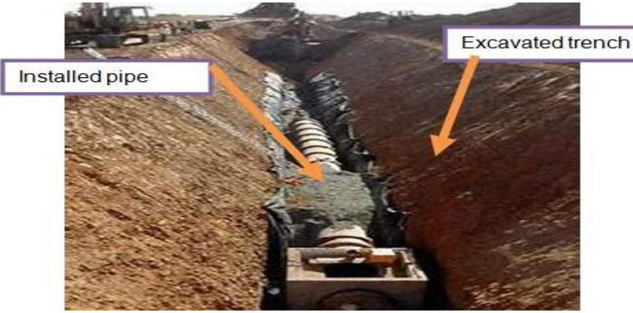
Figure 8: Open excavation
