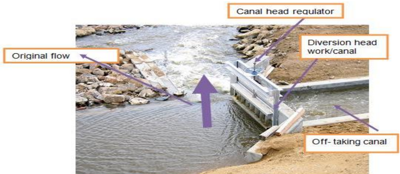
Figure 6: Diversion of river or stream
